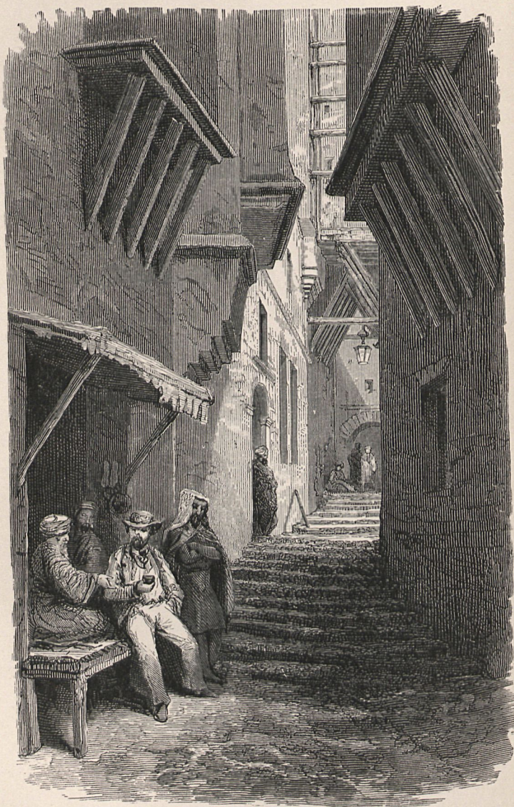
STREET IN ALGIERS.
